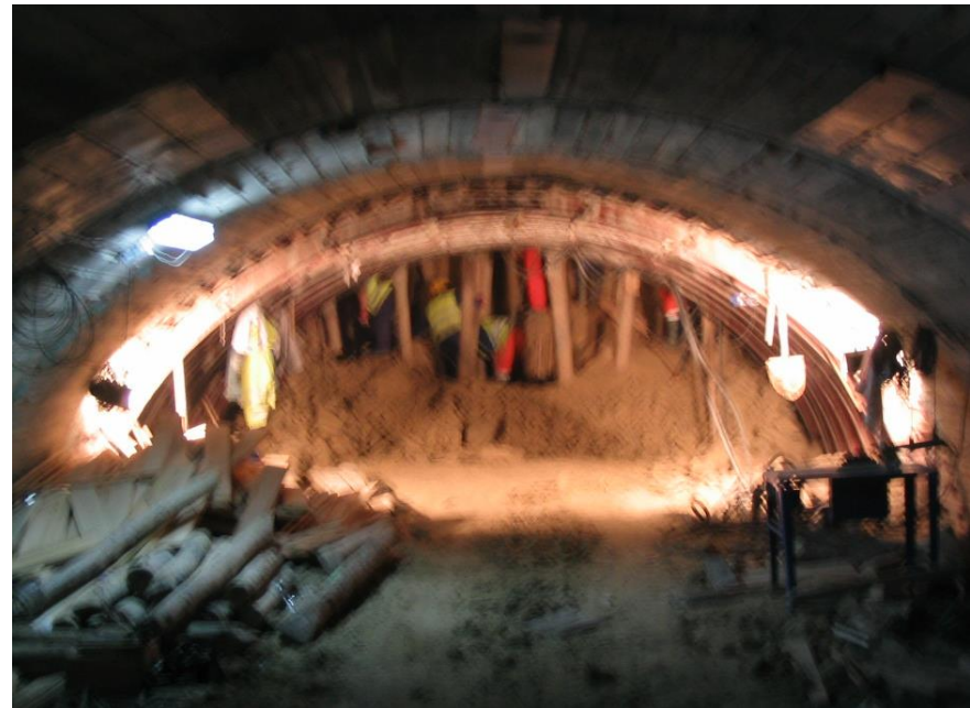
Tunnel- front topheading
