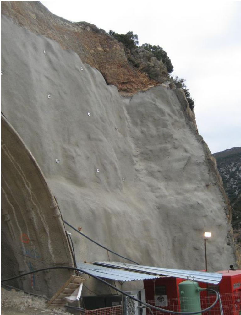
North portal Nueno tunnel
