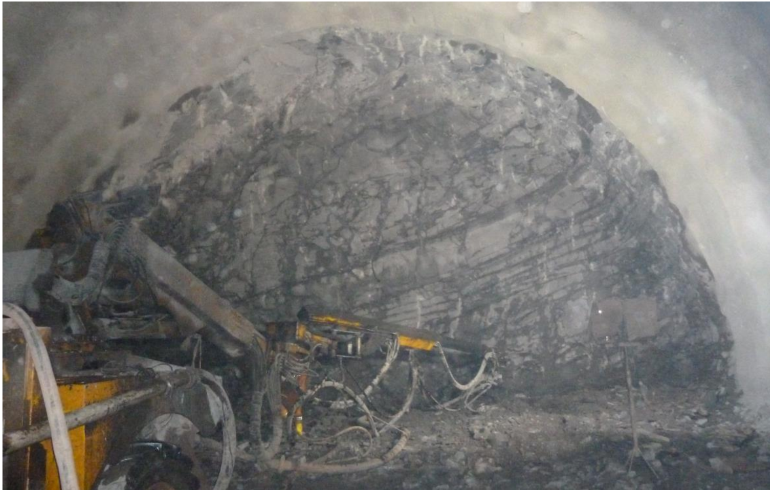
Main tunnel section
