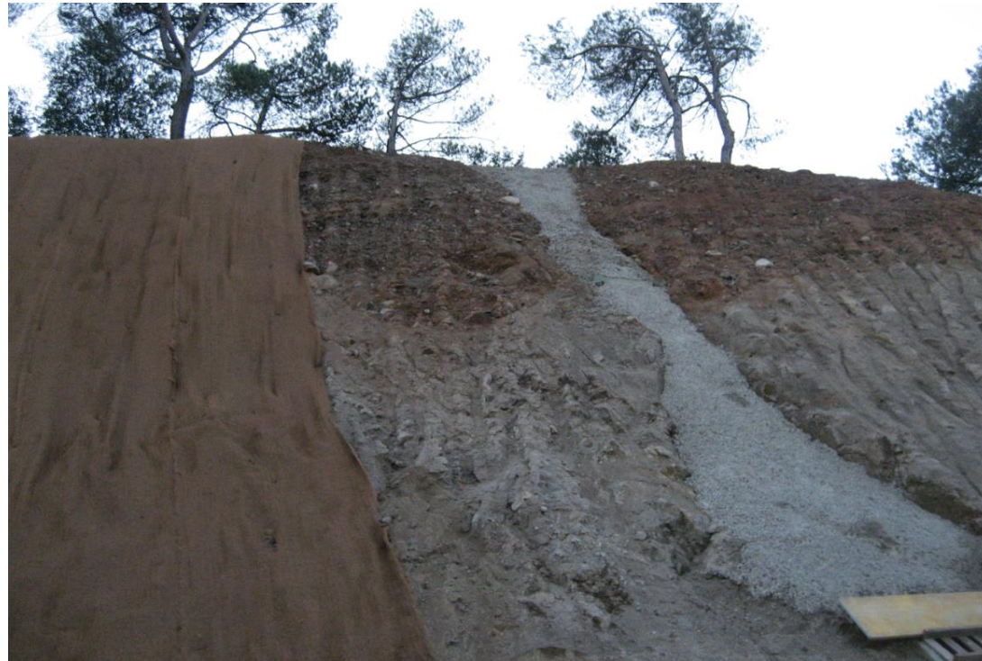
Alforja slopes stability
