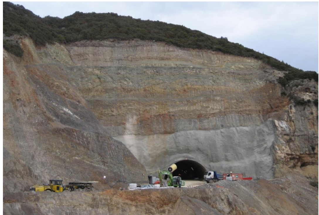
South portal Nueno tunnel
