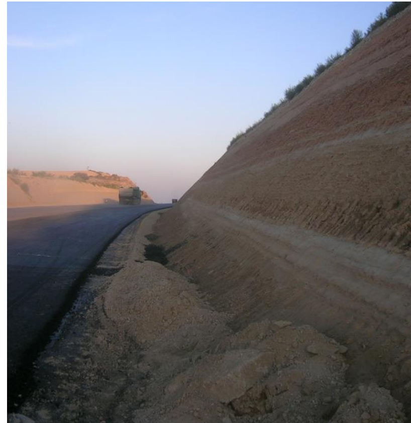
Lleida airport road slopes stability
