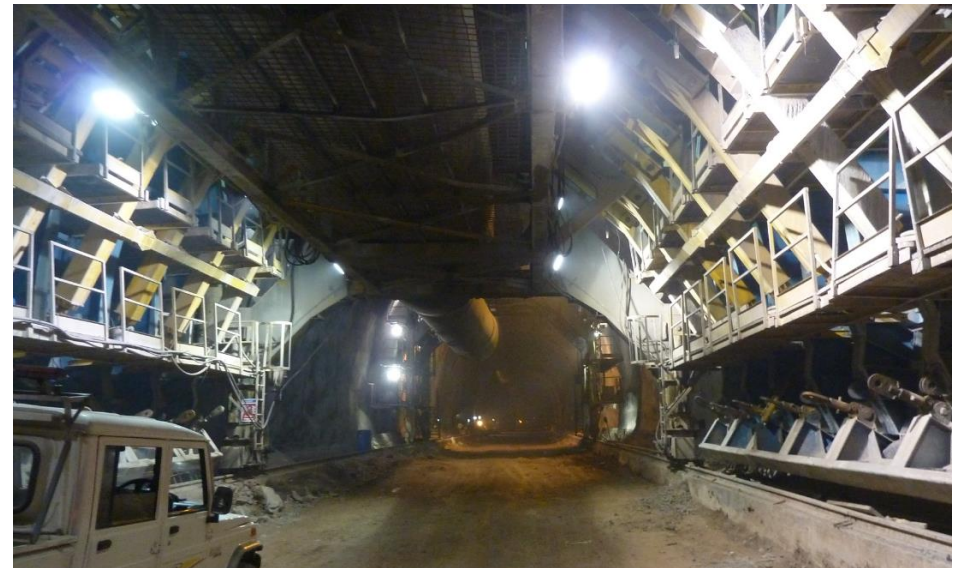
Lay – By final lining
