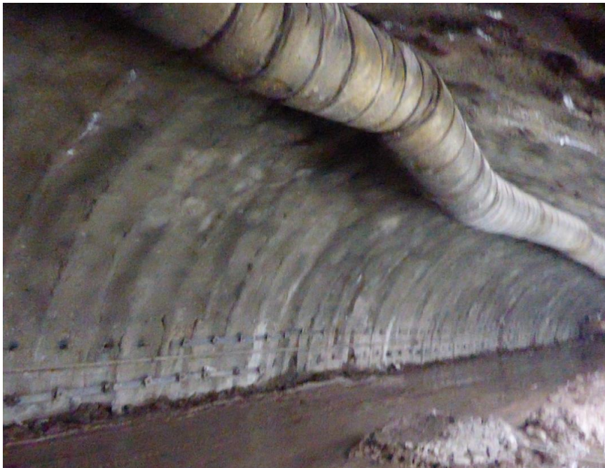
Top heading stretch tunnel 4
