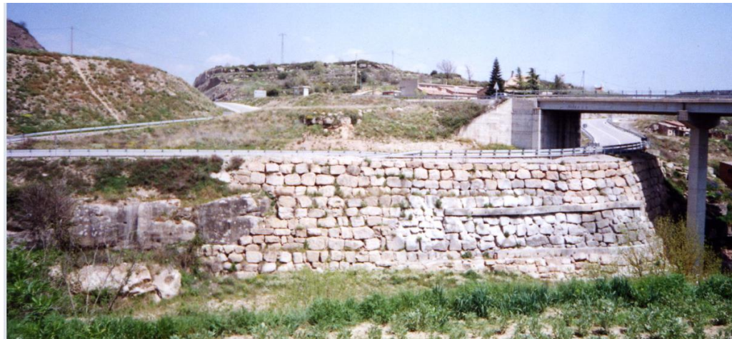
Villadomiu wall reinforcement
