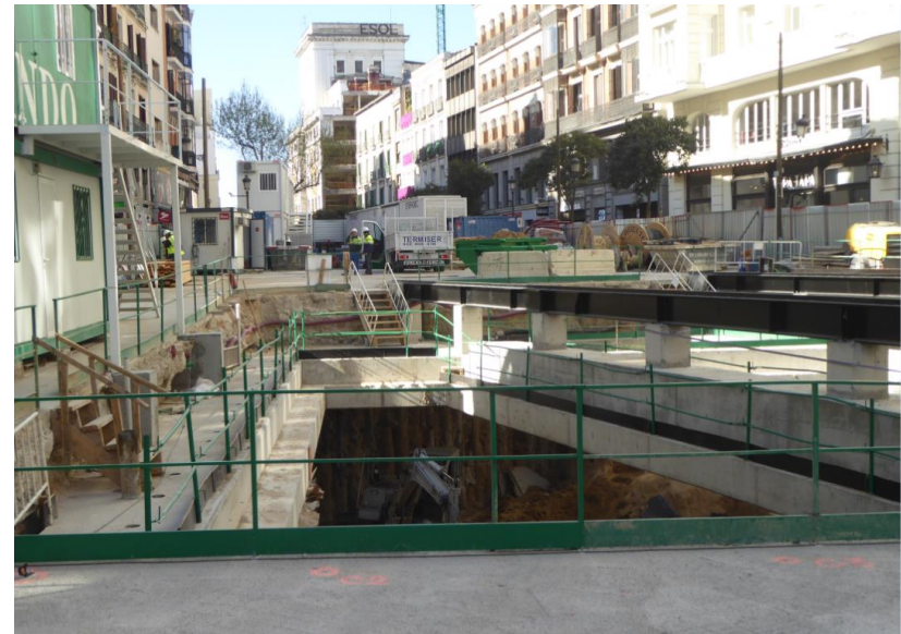
General view slab more beam loading and tied beam
