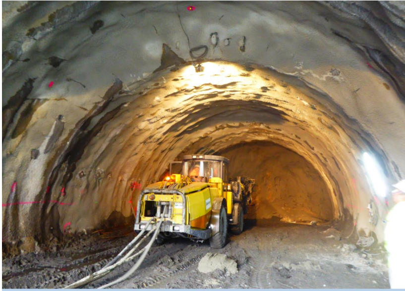
Asymmetric deformed tunnel contour
