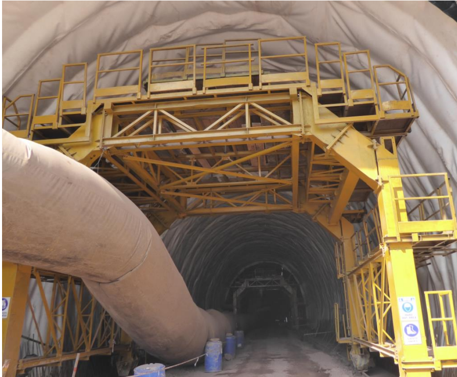
Final lining Carriage Tunnel 1
