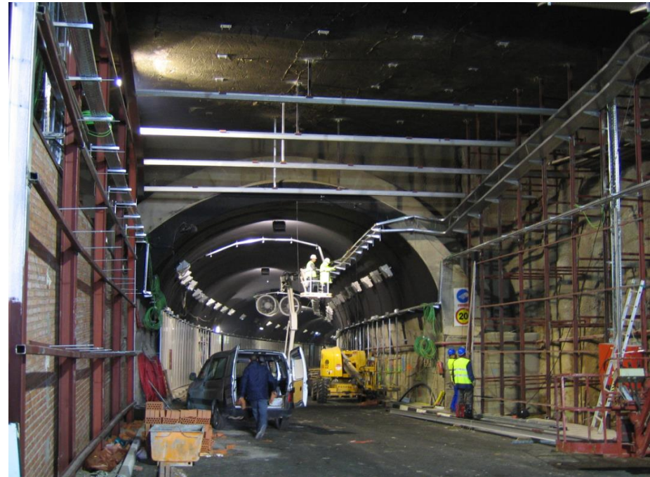
One way two lanes_tunnel
