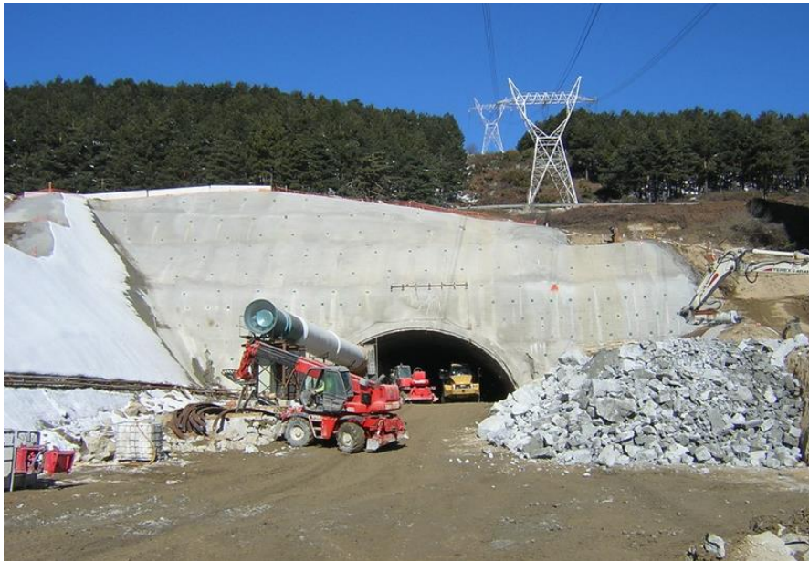
South tunnel portal
