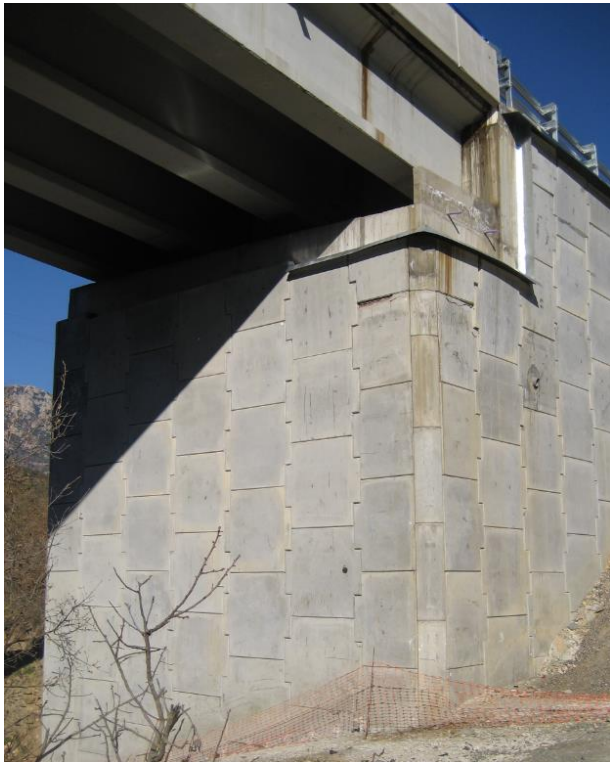
Ager reinforced soil wall
