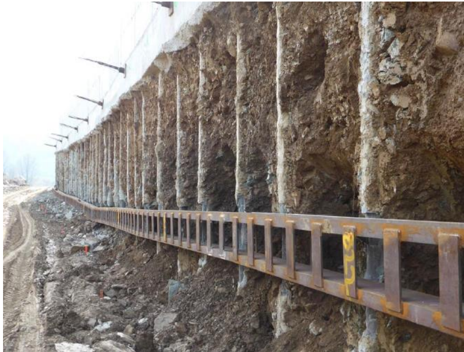
Micropile with longitudinal brace in soil
