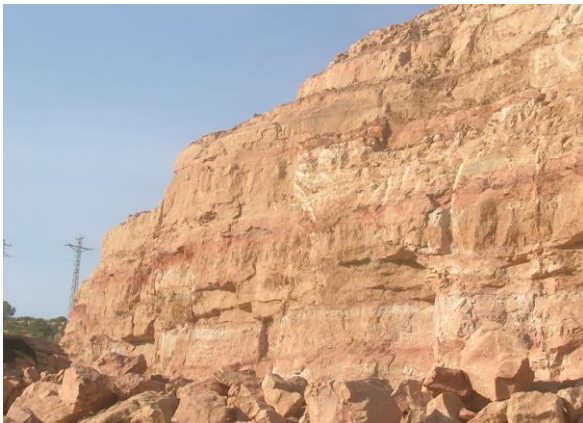
Castaldans slopes stability
