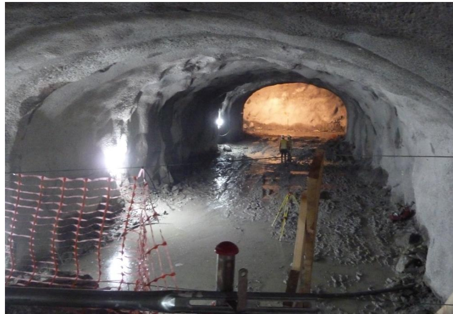
Main tunnel top heading
