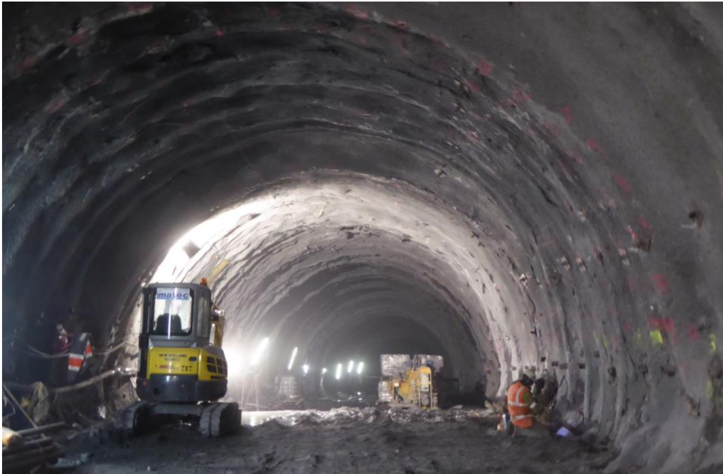
Top_heading_reinforcement_squeezing stretch
