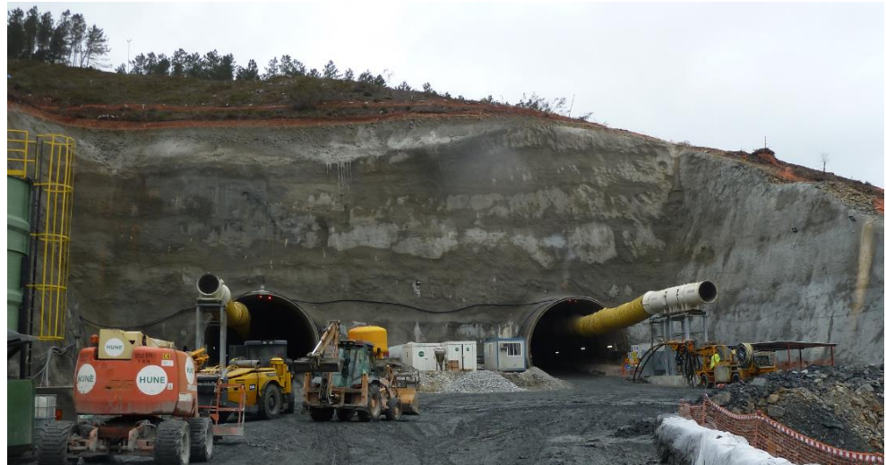
Prado tunnel west portal
