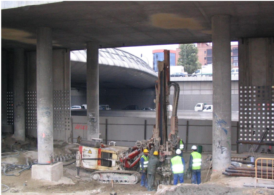
Crossing under M30 highway
