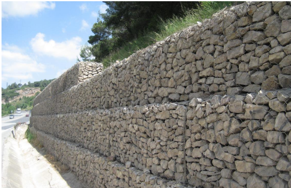
Centelles – Ripoll gabions wall
