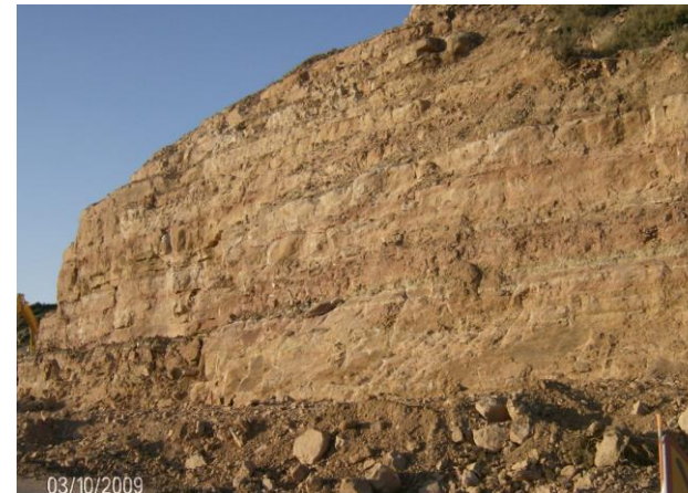
Castaldans slopes stability
