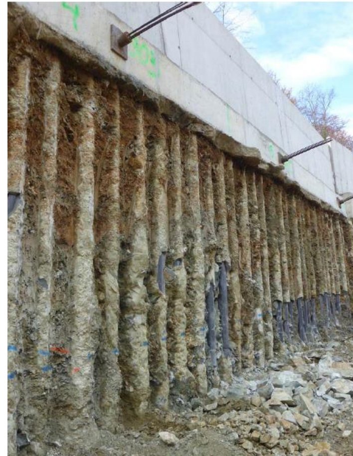
Micropiles sheet due to join with beam
