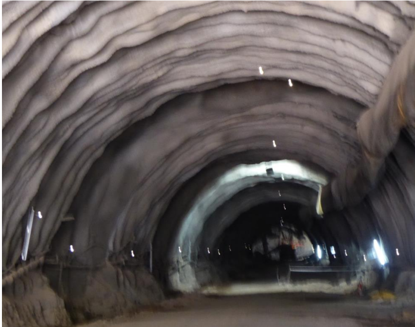
Top heading section tunnel 3
