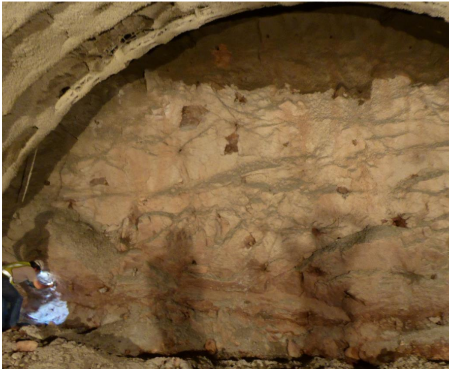
Top heading face tunnel 2
