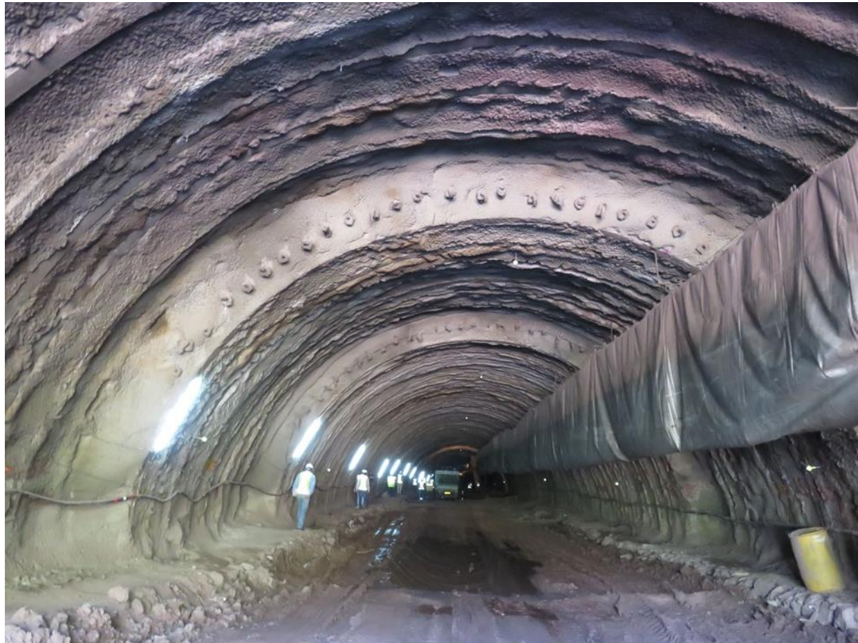
Top heading stretch tunnel 5
