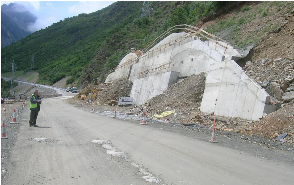
The Bonaigua wall stability
