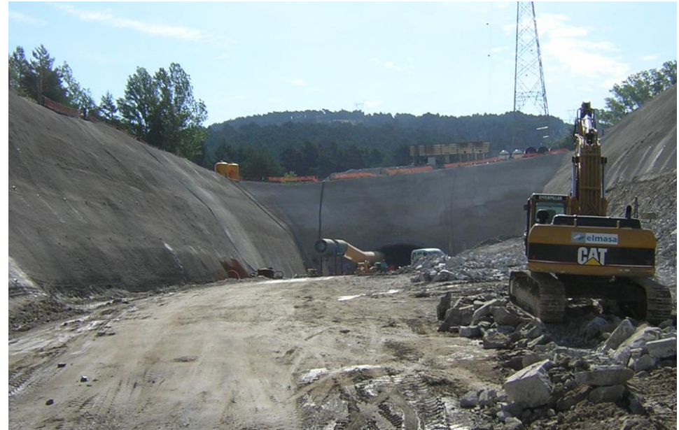
North Tunnel portal
