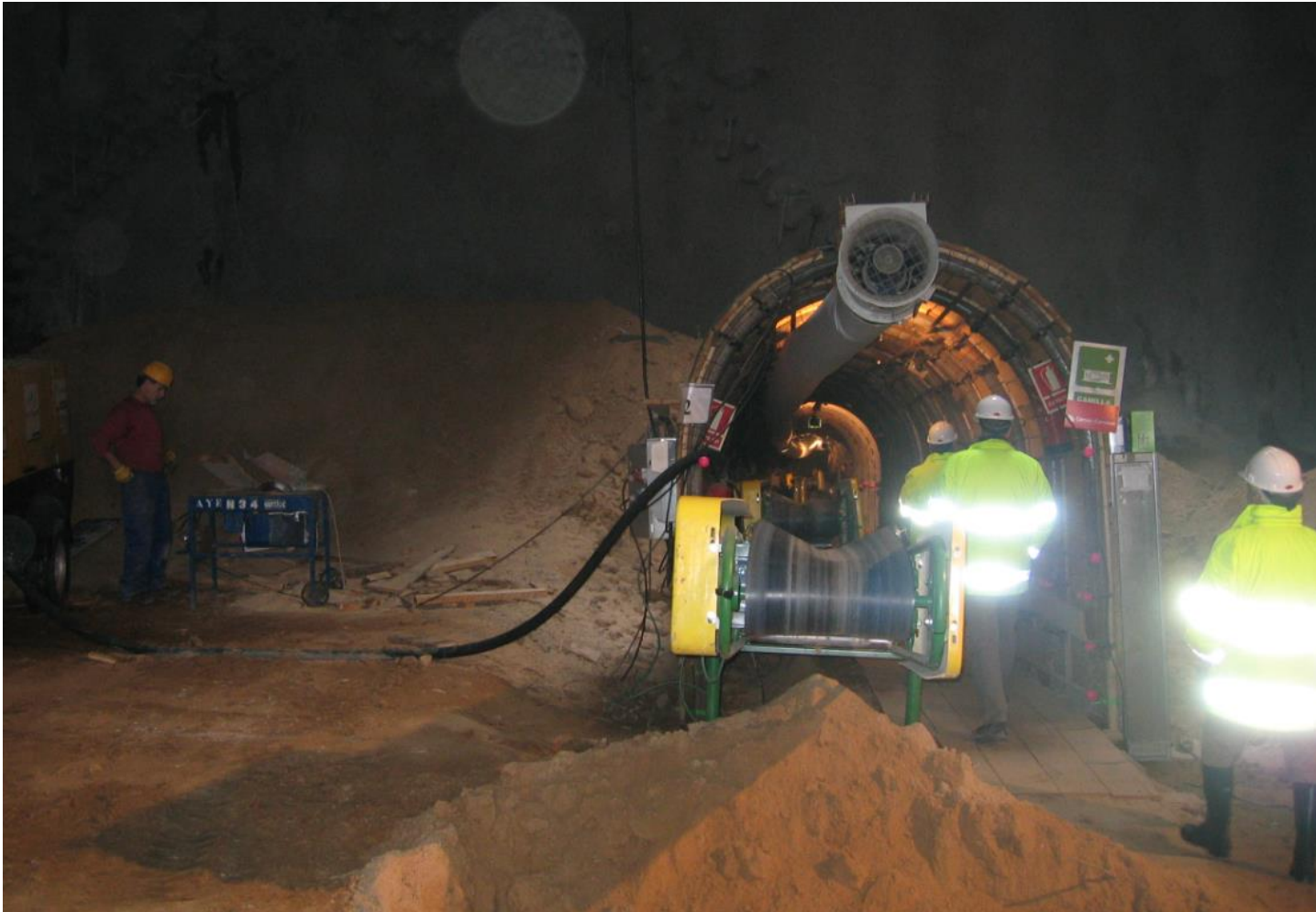
Underground tunnel portal
